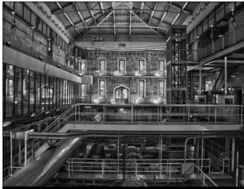
Pumping Station by Jim Beck
